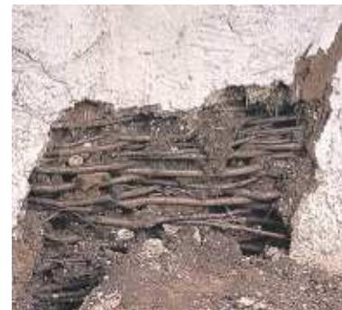
Wattle and daub: basketwork covered with clay.
