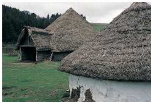
A British farmhouse was circular, thereby minimizing heat loss through the walls, which were usually made of wattle and daub attached to a wooden frame. The steeply sloping thatched roof allowed rain and snow to run off quickly.
