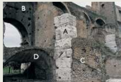
Concrete was used alongside other building materials, as in the Colosseum, above. Top: On the outside the amphitheater appears to be all stone. Bottom: Inside we find a mixture of stone walls (A and B), walls made of brick-faced concrete (C), and concrete vaulting (D).
